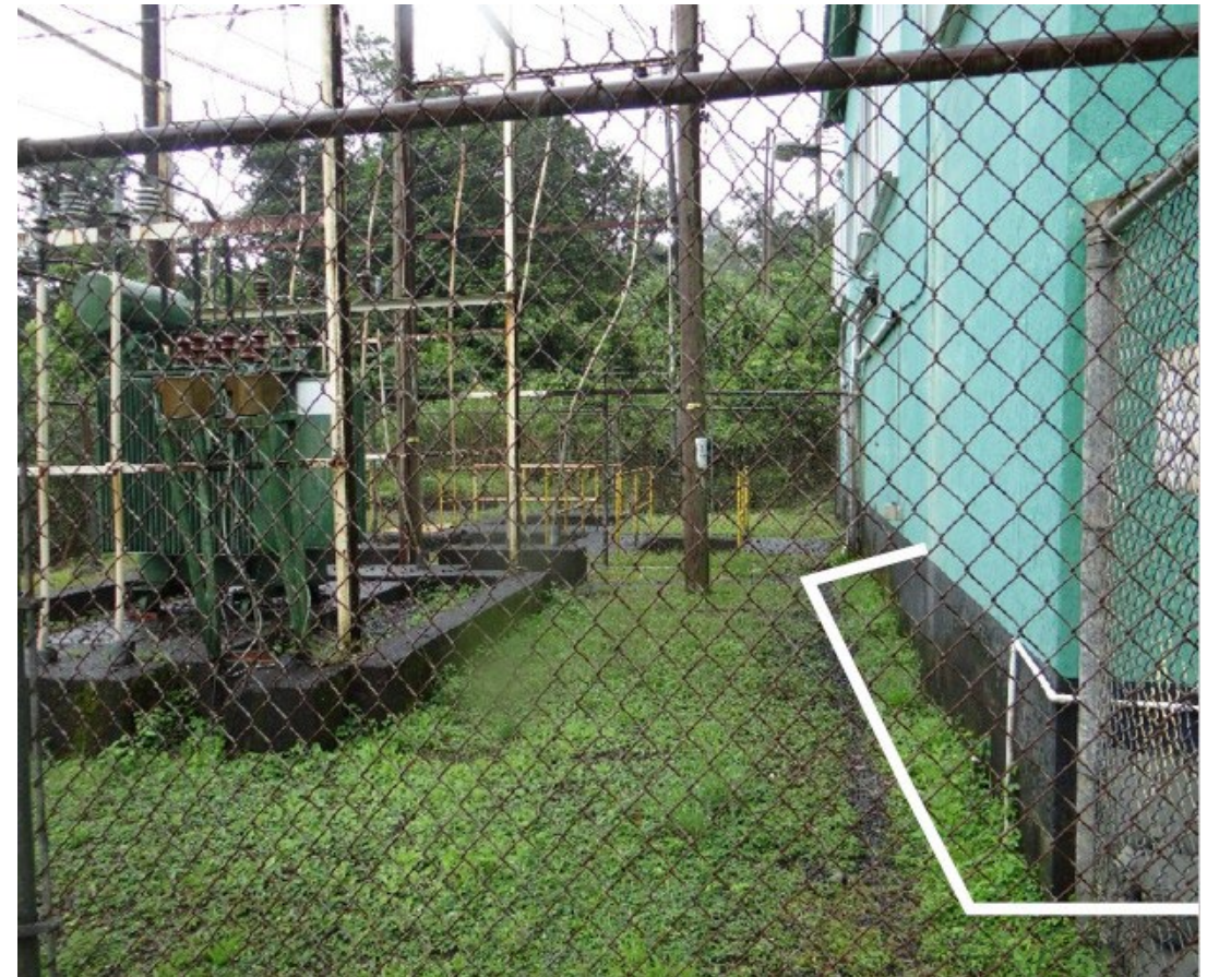
Back side of the Laudat power station building
