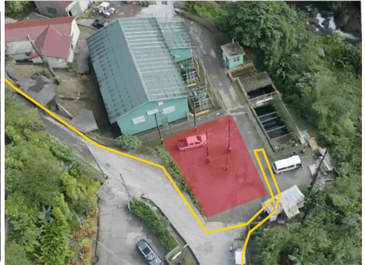
Aerial view of Trafalgar power station and new SS location
