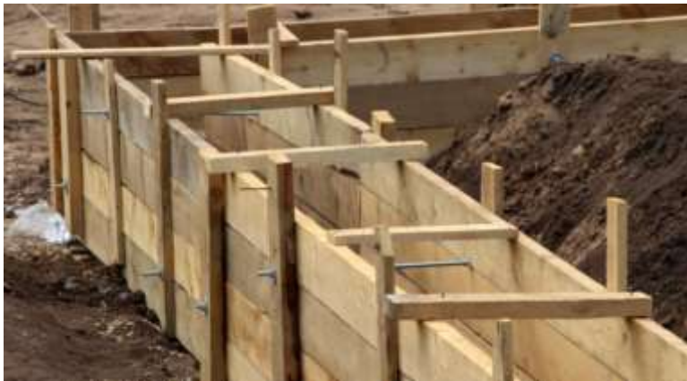
Figure 12: Ordinary system formwork (Type 1)
