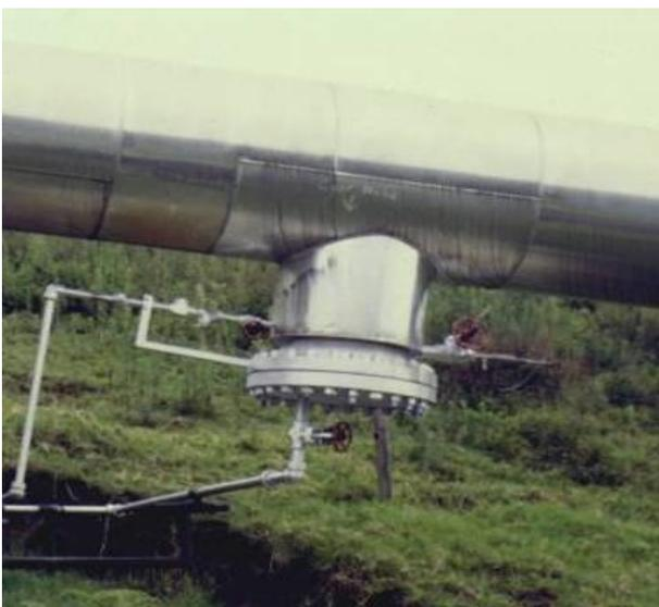
**Figure 4-12: Condensate collection drain pot (CDP)**
