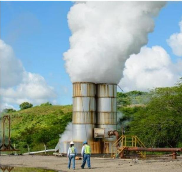
Figure 4-9: Atmospheric Flash Tank (AFT / Silencer)
