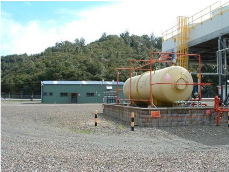
Figure 4-17: Working Fluid Storage Tank with bunding and fire protection system (red piping)
