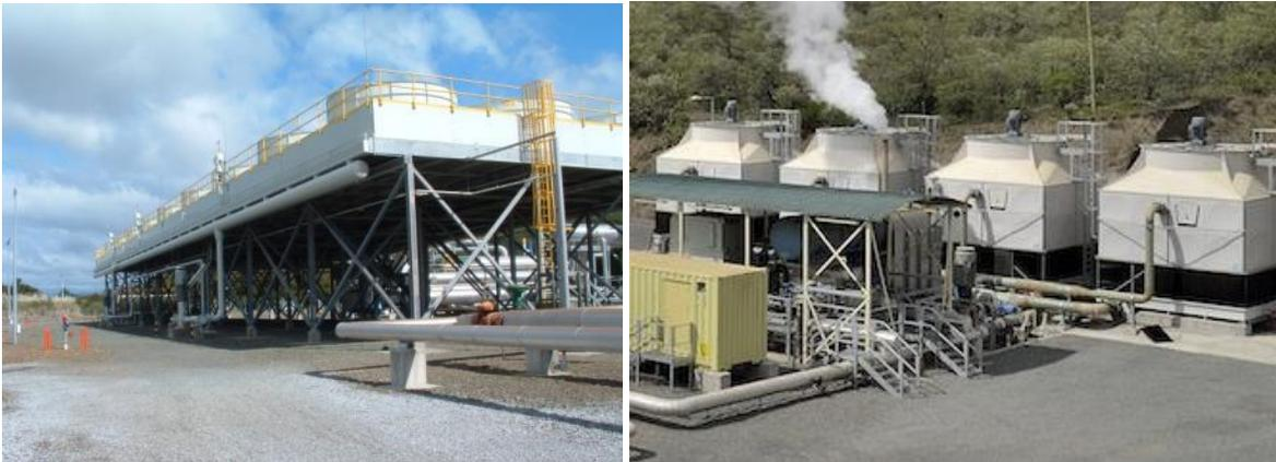
Figure 4-7: Air cooling for 9MW<sub>e</sub> binary plant (left). Evaporative cooling tower for 5MW<sub>e</sub> plant (right)
