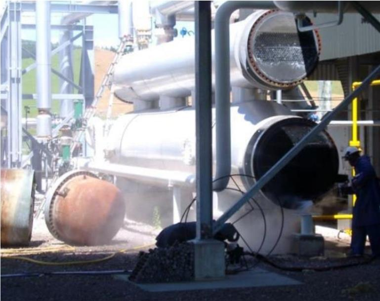
Figure 4-6: Binary plant heat exchangers (large plant example)
