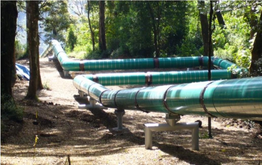
**Figure 4-16: Typical pipe expansion loop (large steam line, under construction)**
