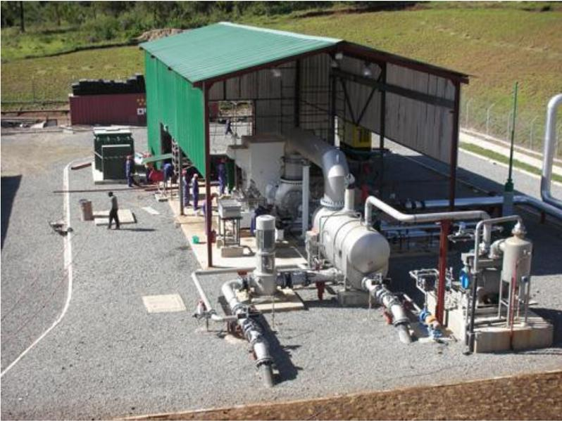
Figure 4-4: Condensing Steam Turbine (Source: GDA - <http://www.gdareno.com>)
