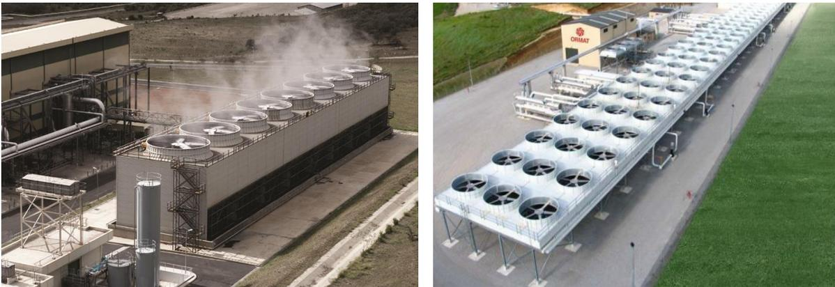
Figure 3-1: Turbine Hall and Evaporative Cooling Tower (left). Air cooling for 20MW plant (right)
