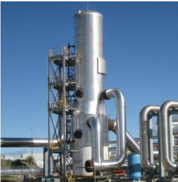
**Figure 4-8: Typical geothermal separator**
