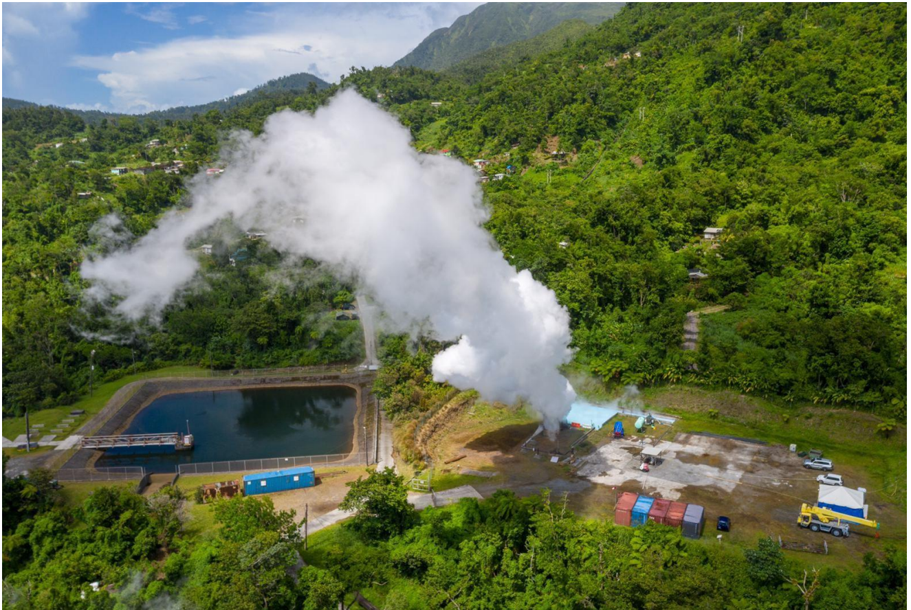
Photo No. 4. Existing brine pond and well pad during flow test of WW-P1 and WW-03
