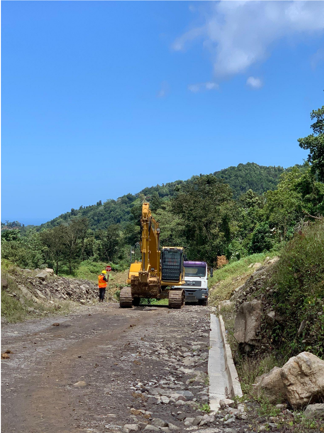
Photo No. 3. Grading works at the Project site
