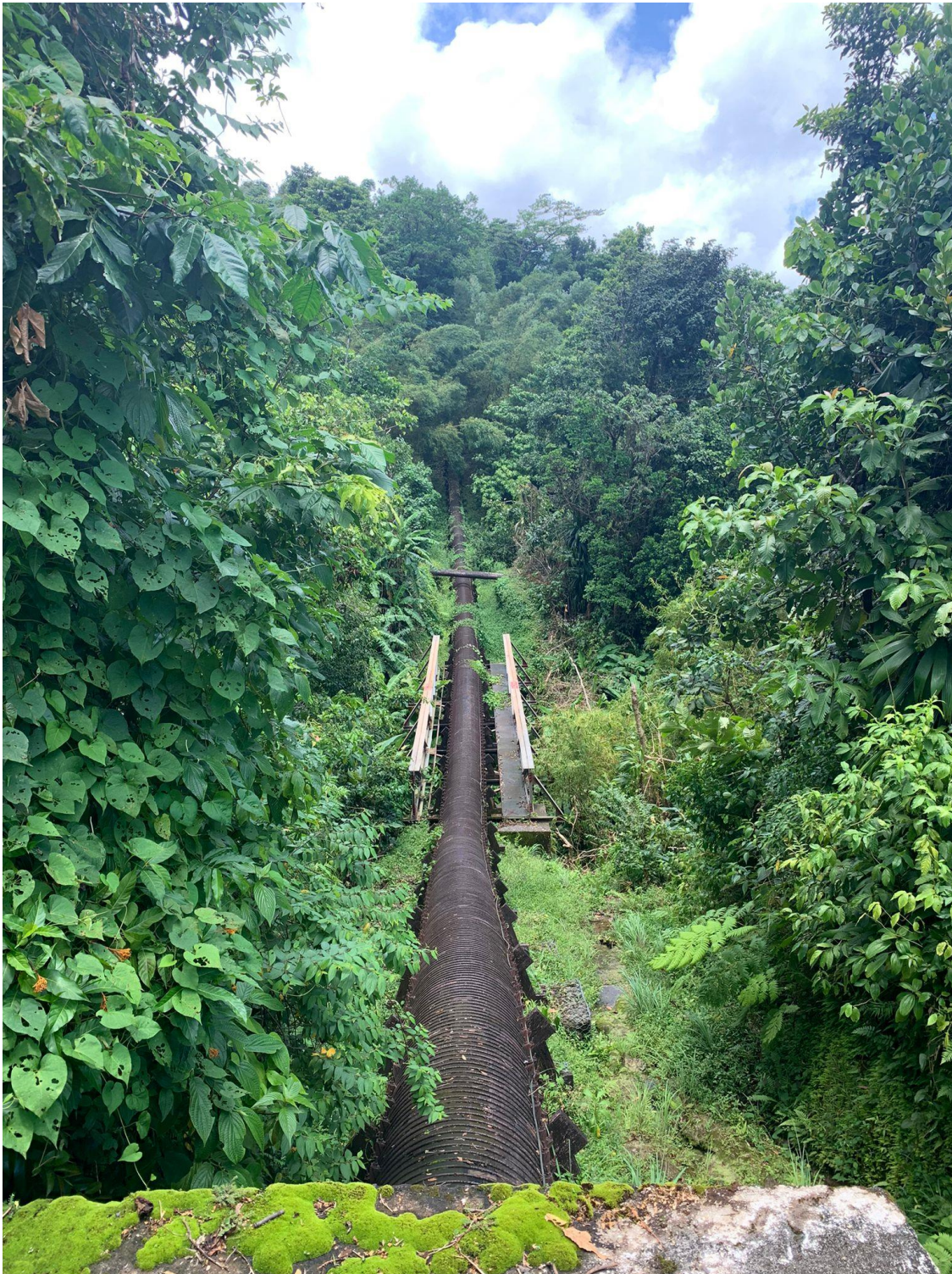
Photo No. 2 – Right of Way of the injection pipeline
